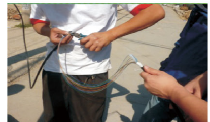
In-situ branching of slotted-core tight buffered optical cable
